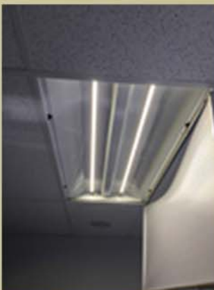
Troffer LED strips installed
