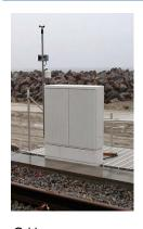
The cubicle cabinet is an important protective part of the system. The cabinet is designed for the demanding requirement in the out door railway environment. The cabinet is installed on DIN sized base, made from the same material.
